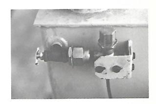
Mounted on the top of the tank is the pressure relief valve which opens when pressure in the tank reaches 14-16 PSI. Pressure can increase since, at low fluid levels, pressure is maintained at 6 PSI and, when the fluid level raises, the air in the tank is compressed. If the pressure was not relieved, the tank would bulge or burst.
